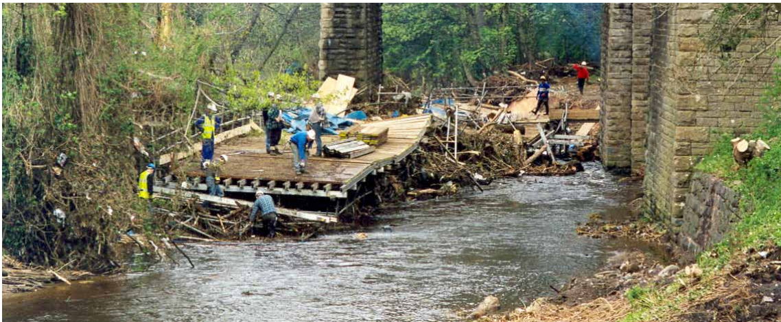
Figure 11: Large woody debris trapped at a bridge. Photograph courtesy of the City of Edinburgh Council.
