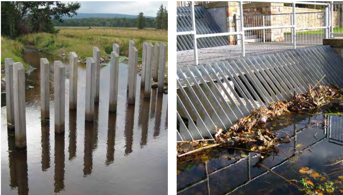
Figure 47: Trash screen bar spacing should be as large as possible (see photo on left). Smaller bar spacing can create a barrier to fish passage (see photo on right).
