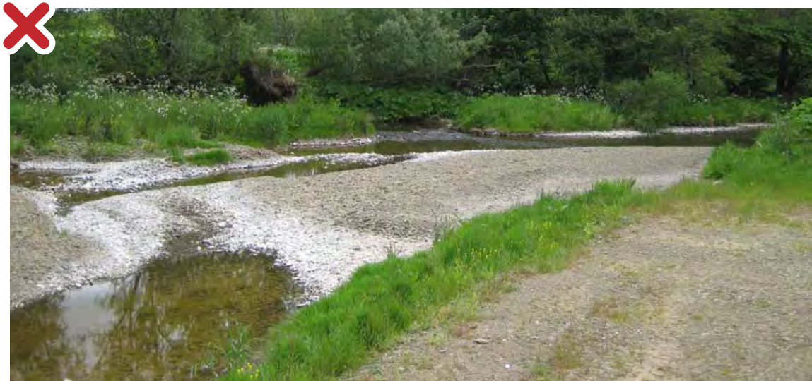
Figure 25: Poor practice, do not locate crossings on depositional areas. Indicators of a depositional area include gravel bars.
