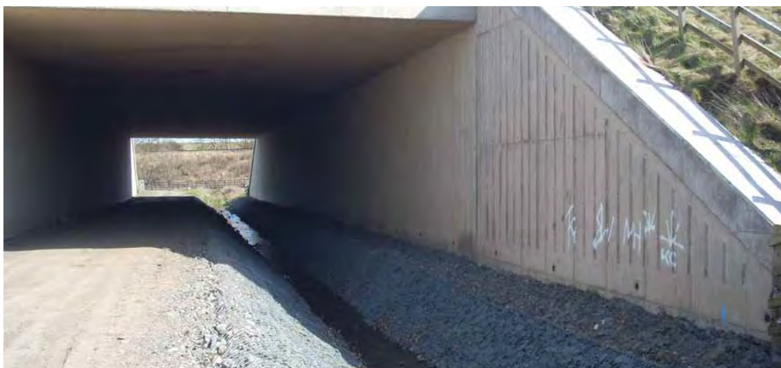
Figure 37: Longer crossings may lack light and moisture which can prevent the establishment of vegetation under the crossing and weaken the banks. This may result in the requirement for bank reinforcement however the natural bed should still be maintained.
