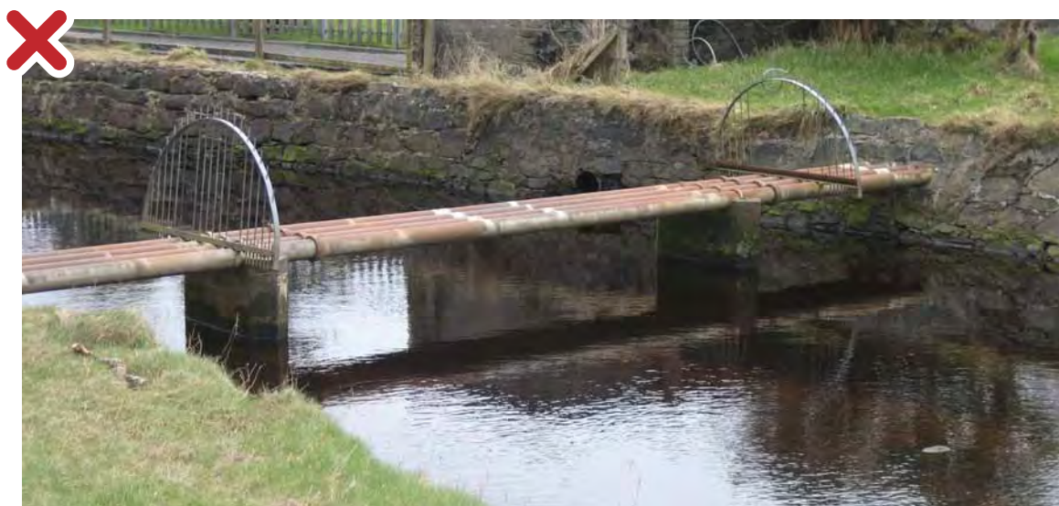
Figure 55: Poor practice, pipeline laid in the river channel. Can cause scour around the structure and pipe is at risk of damage during high flows.
