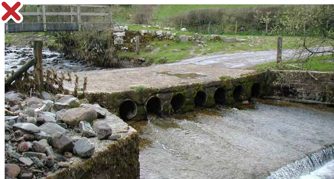
Figure 6: Poor practice. Pipe bridge creating a barrier to fish passage, showing a drop from the invert to the riverbed (perched). Undersized pipes are too small and dark for fish to enter and in high flows water may be too fast for fish to swim against.
