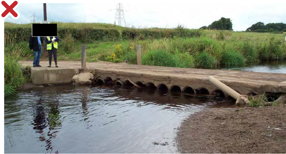
Figure 6: Poor practice. Pipe bridge creating a barrier to fish passage, showing a drop from the invert to the riverbed (perched). Undersized pipes are too small and dark for fish to enter and in high flows water may be too fast for fish to swim against.
